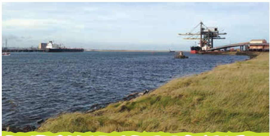
View of current frontage where proposed quay will be constructed
